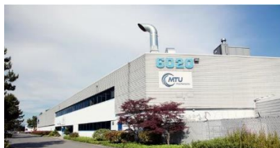
MTU Maintenance Canada
