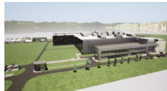
MTU Maintenance Serbia Opening October 2022
