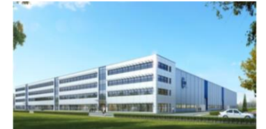
MTU Maintenance Zhuhai (JV) Shop expansion 2021
