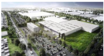
MTU Maintenance Hannover Shop expansion 2021
