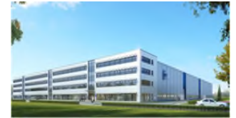
MTU Maintenance Zhuhai (JV) Shop expansion 2021
