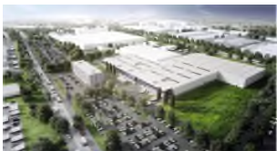
MTU Maintenance Hannover Shop expansion 2021
