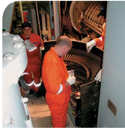
A stator case is removed on-site by MTU's field service team.
