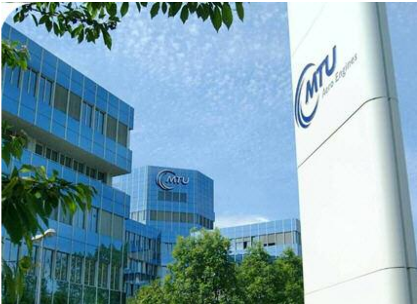
MTU Aero Engines, Munich Companies headquarters
