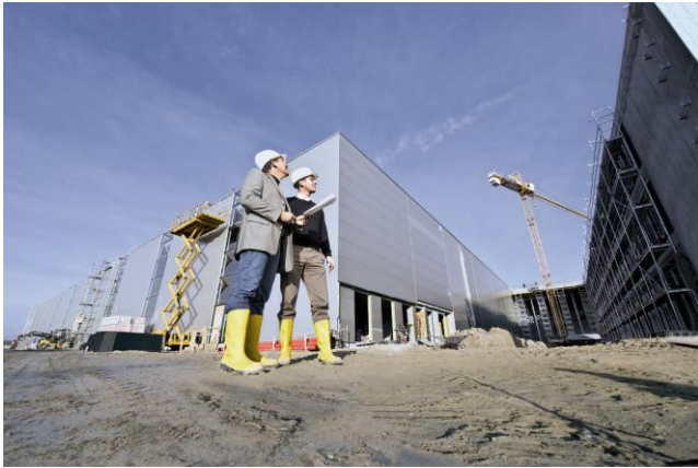
F1: Construction phase in Rzeszów (source: MTU Aero Engines)
